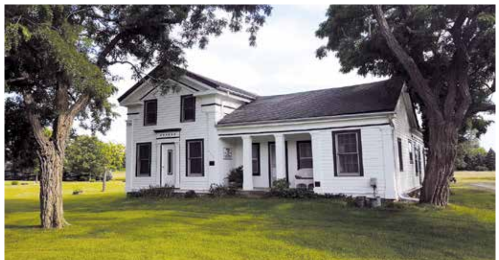
Warner Homestead, Brighton Township, Livingston County (Region 9). Photo: Tim Bennett
