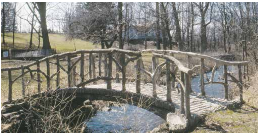
McCourtie Park, Somerset Center: In the 1920s, Mexican folk artists George Cardosa and Ralph Corona were hired by business man W.H.L McCourtie to build a series of trabajo rustico structures on his estate. They created bridges and birdhouses using the technique in which wet concrete is shaped to look like faux wood. Now a public park, it was listed in the National Register of Historic Places in 1992.
