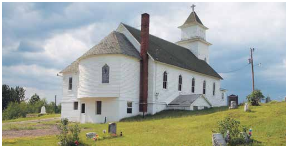
St. Henry's Evangelical Lutheran Church and Cemetery reflects the long Finnish American heritage in the Nisula area in Houghton County's Laird Township and, more broadly, in the western Upper Peninsula of Michigan.
